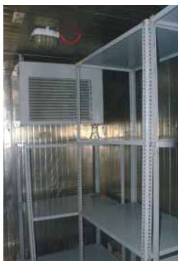
Non functioning WIC at SVS
