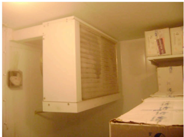
WIF (3), Alternate use of cooling unit
