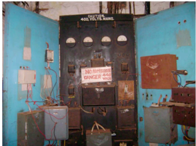
Central electric distribution unit
