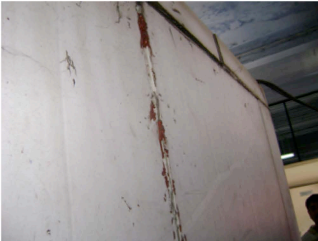
WIF (2), formation of cracks, signs of repair attempts earlier
