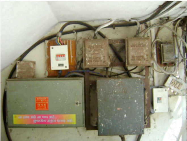
Main electric board of building
