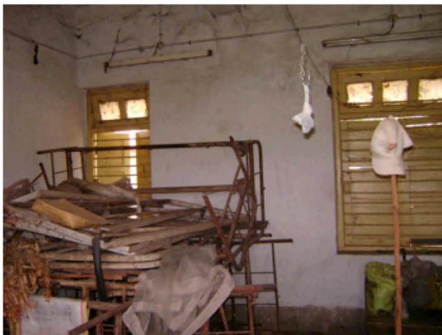
Room proposed for generator
