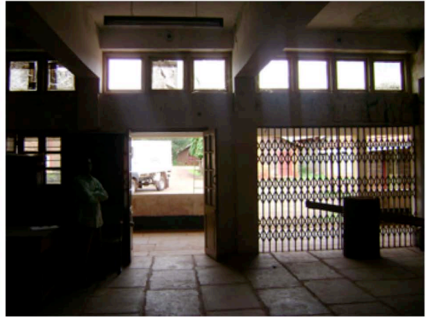
View of main gate from inside
