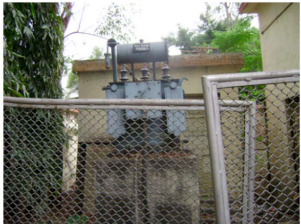
Electric Transformer inside campus
