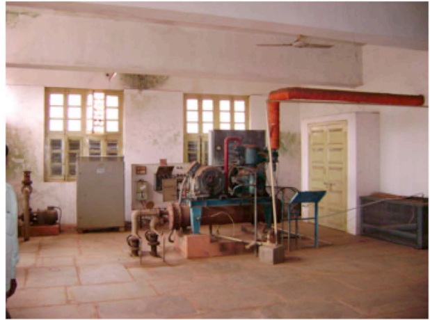
AC plant installed at the site
