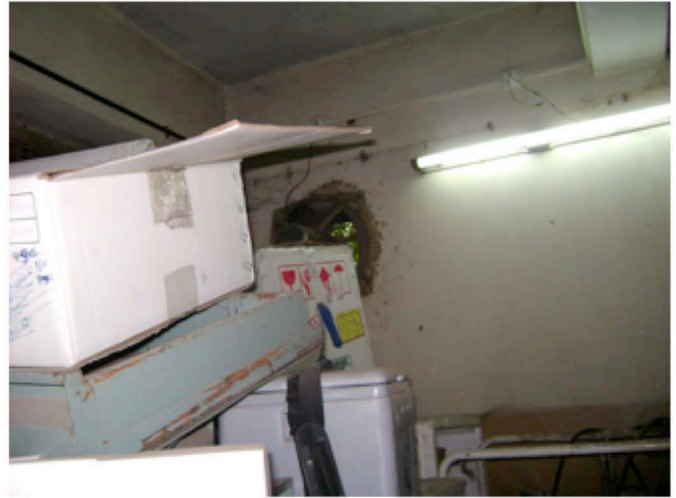
Extractor fan installed in stabilizer room
