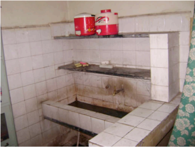
Water sink and washing room
