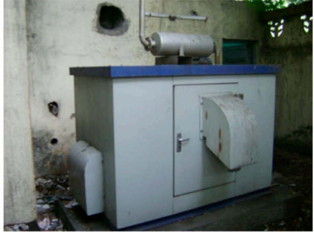
Installed generator for existing WIC
