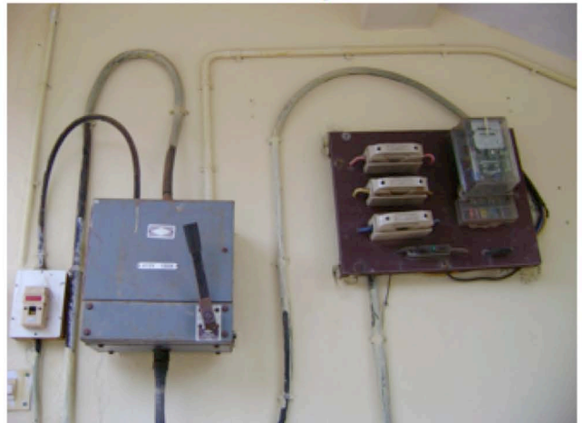
Main fuse and meter of building
