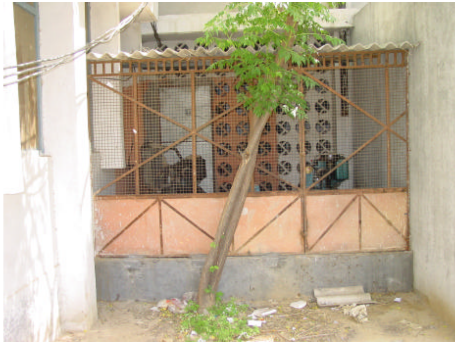
Proposed room for installation of generator for WIF. Facility is well protected and well ventilated.
