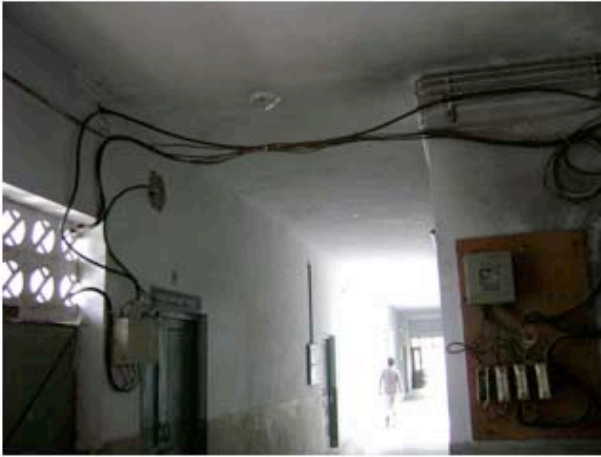
Poor quality of electrical installation
