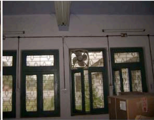
Extractor fan installed, location "A"
