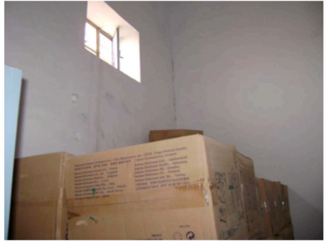
Room proposed for generator
