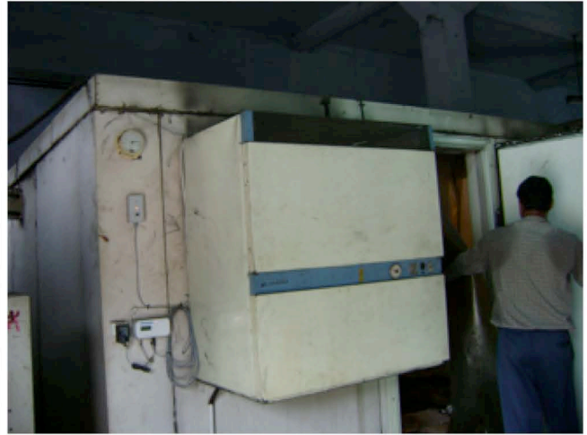
WIF (2) in poor state, refurbishment not recommended
