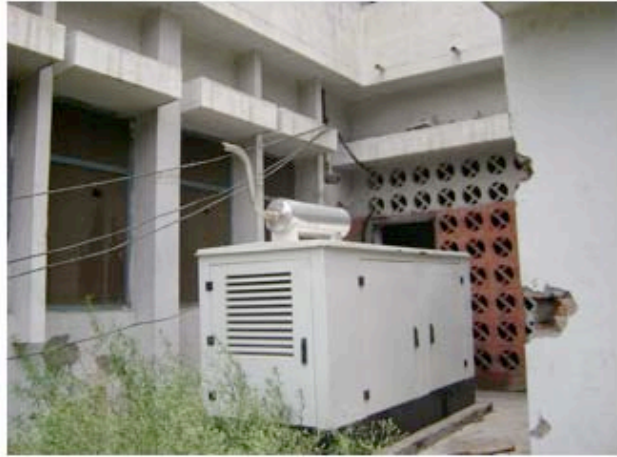
Installed generator
