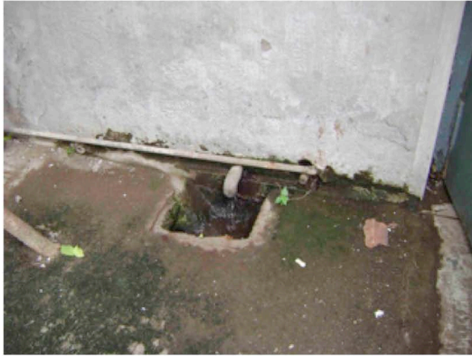
Underground drainage system
