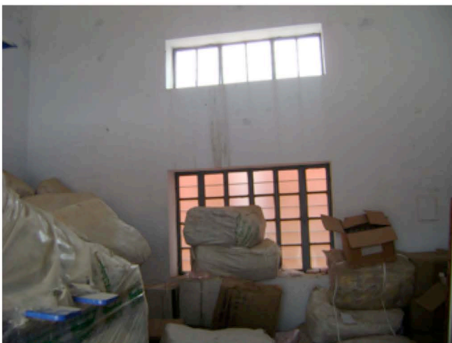
Ventilation and lighting provisions
