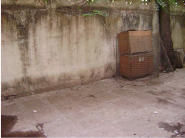
Proposed site for new generator
