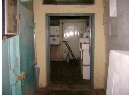
Entrance to installed WIC. Path to this WIC will get constrained after installation of new WIC
