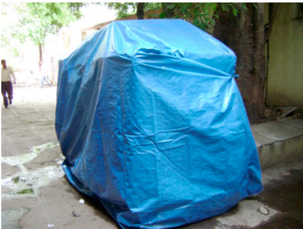
New generator covered and stocked
