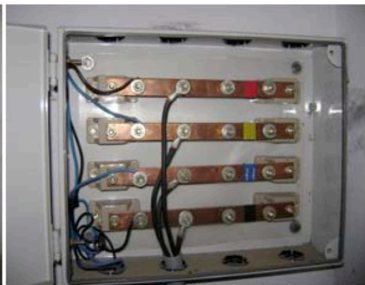
Connections inside electrical panel
