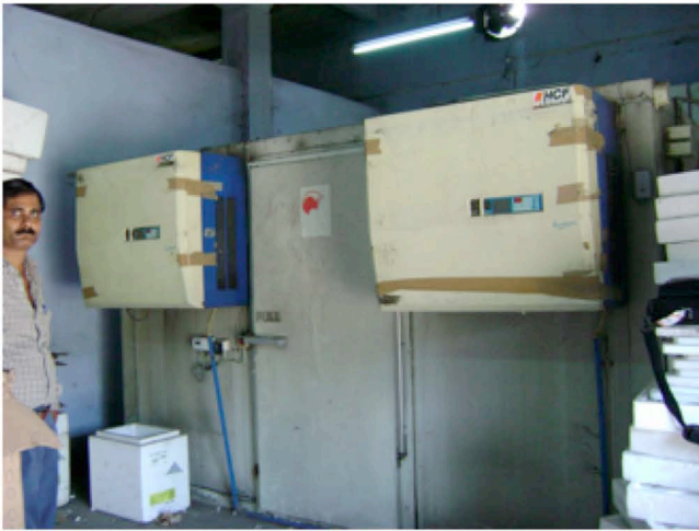
WIF (1) in good shape, cooling units to be replaced
