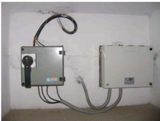
Electrical panel installed, location "A"
