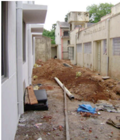
Proposed site for generator
