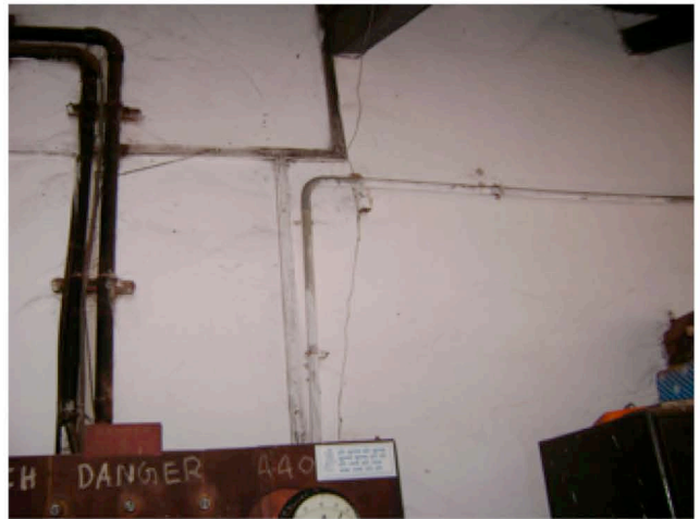
Old electrical wiring at electric hub
