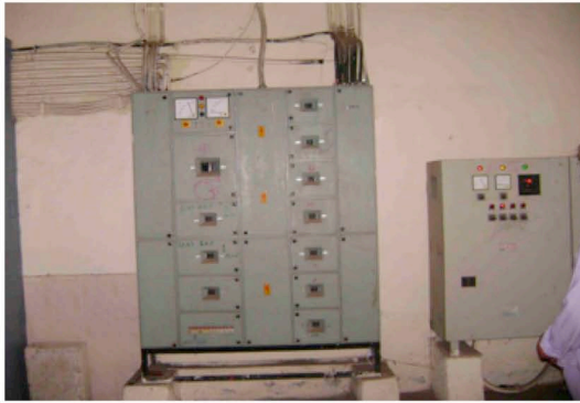
Main power distribution box of building
