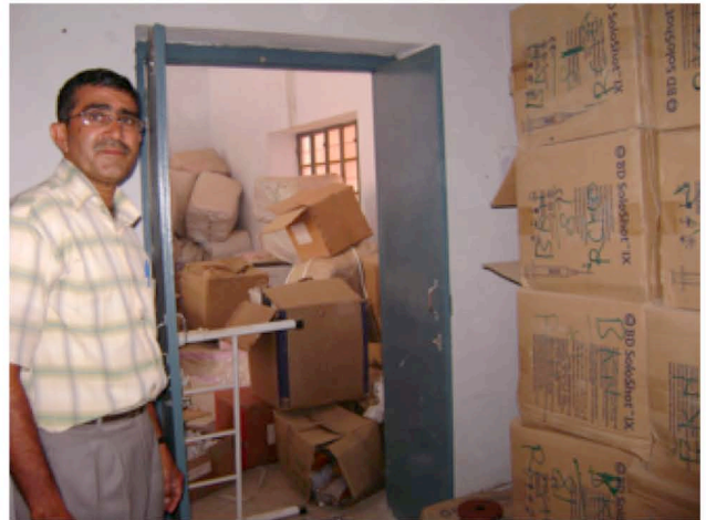
Door leading to generator room
