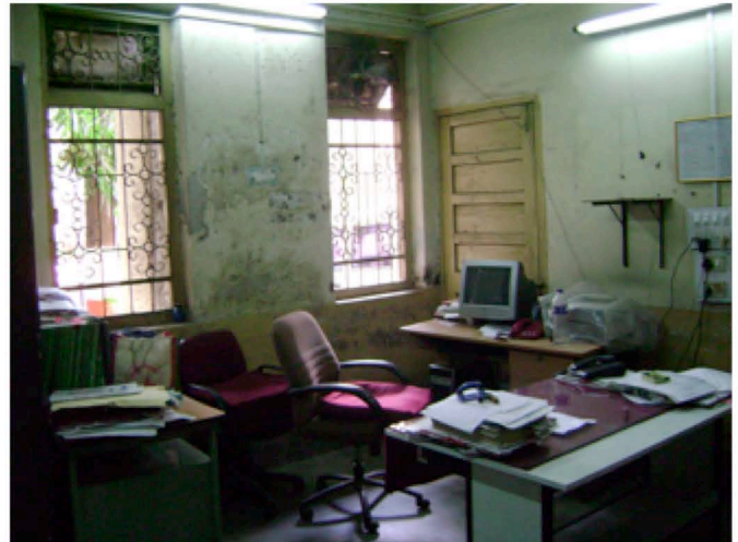
Present storekeeper's office, wall with a door should be demolished for WIF
