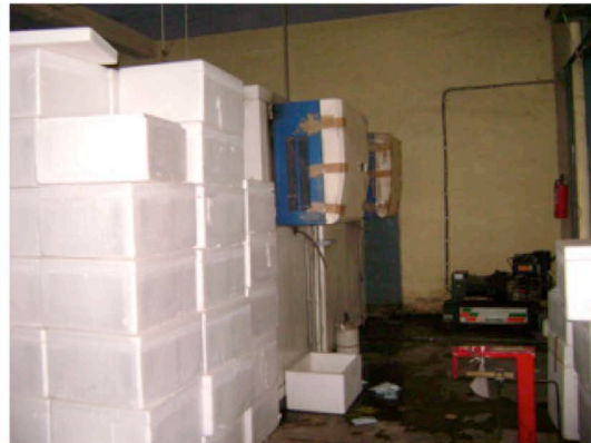
WIF, generator and poor drainage
