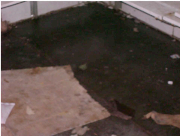
Almost damaged floor of WIF (2)
