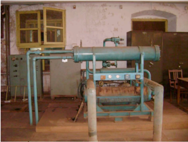
Chiller plant installed at the site
