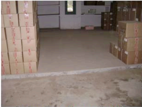
Platform created for mounting WIC, location "A"
