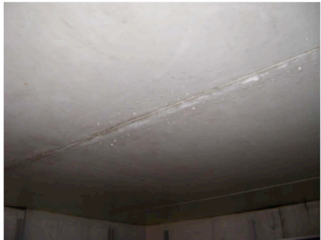
WIF (2), water leaking from ceiling
