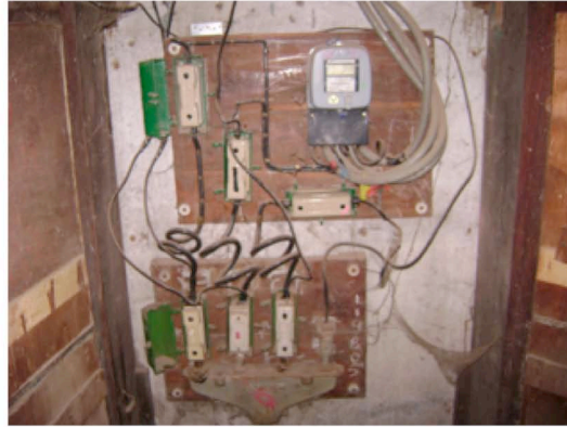
Main fuse board with meter
