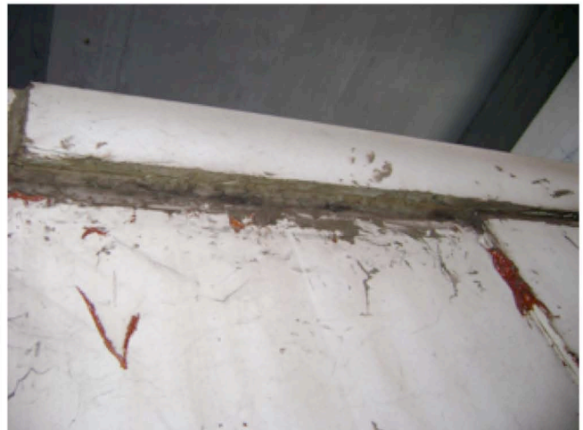
WIF (2), formation of cracks, signs of repair attempts earlier
