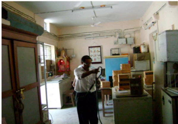
Present refrigeration workshop
