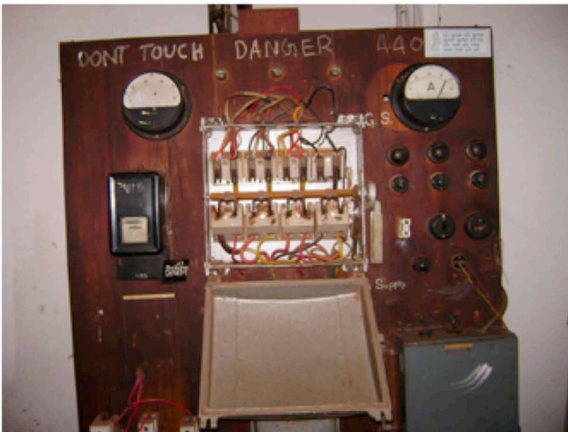
Electric panel of existing cold rooms
