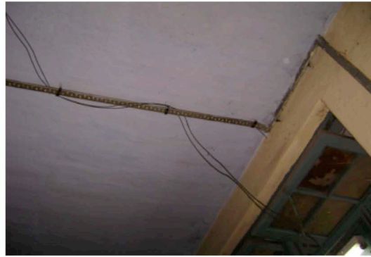
Poor electrical connection to WIF
