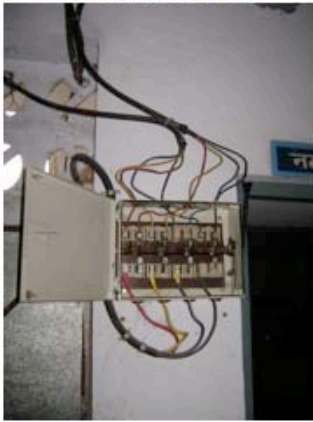
Genset & grid change over switch
