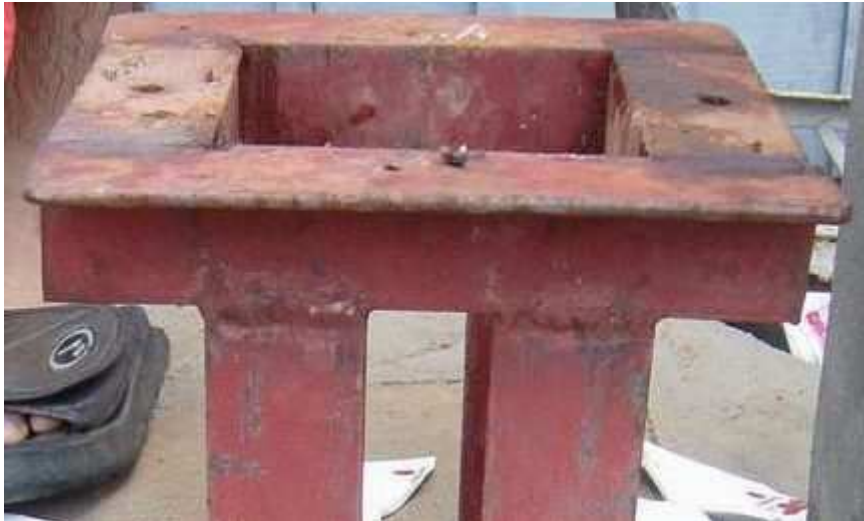
Detail crusher foot top ^
