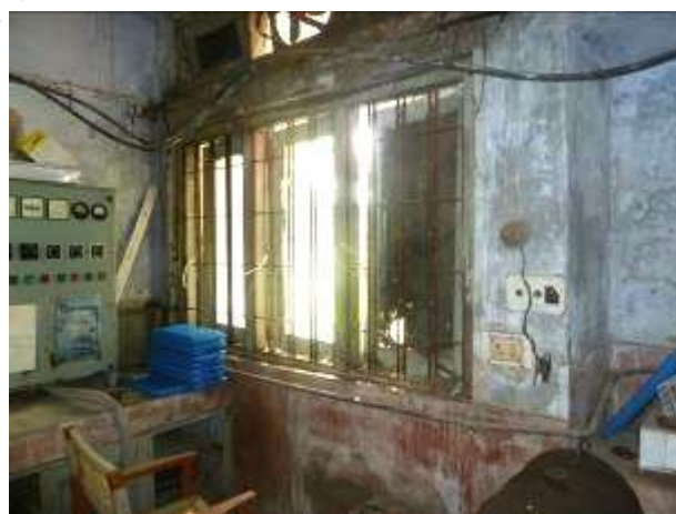
Broken windowpanes at the SVS Gandhinagar
