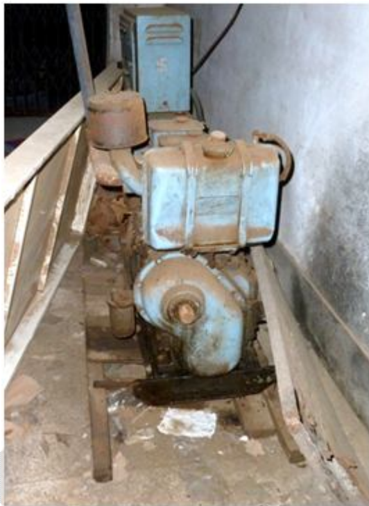
Generator at a DVS before
