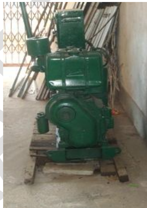
Same Generator after 1 month
