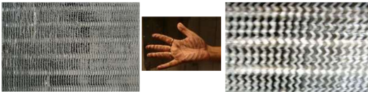
The condition of WIC Condenser before (left) and after (right) servicing at SVS, Pune
