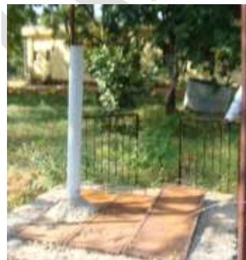
Disposal Pit PHC Shankarpur not in use
