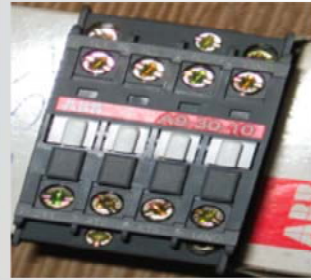
Compressor contactor Code: 0854 HUURRE cold room
