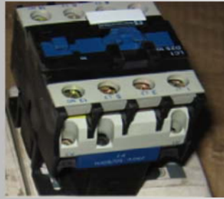
Contactor K-2: Code 0094 HUURRE cold room
