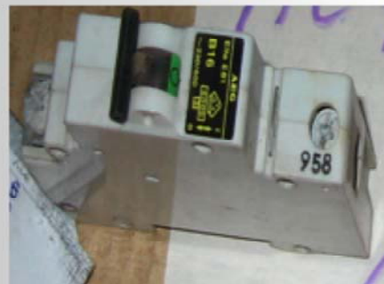
Circuit breaker : Code 0340 HUURRE/FOSTER cold room
