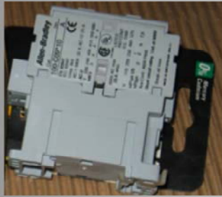
Contactor K-1: Code 0093 HUURRE cold room
