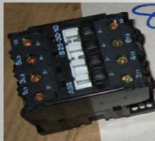
Main contactor : Code 0156 FOSTER cold room
